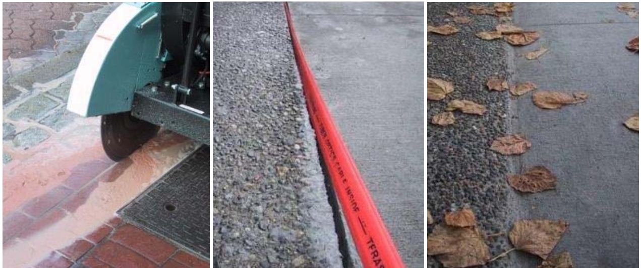
Figure 11 – Example of vertical in-laid Fibre using micro-trenching technique (Source: Teraspan Networks)
