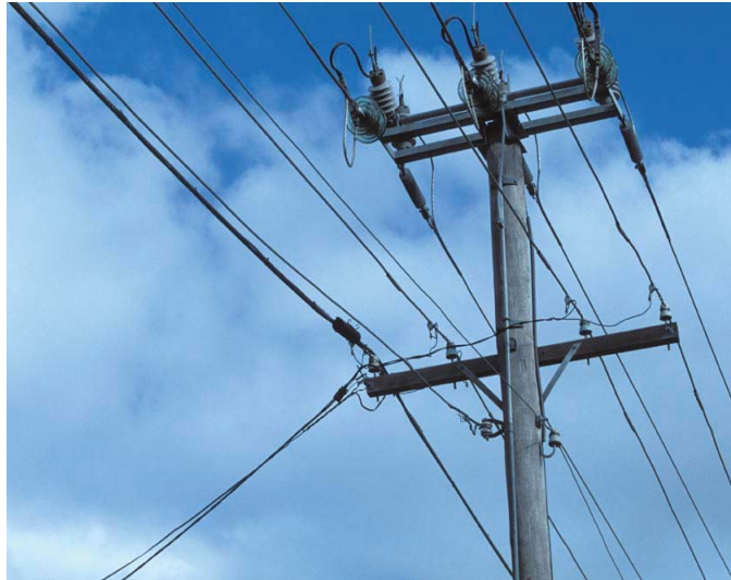
Figure 10 - Low Impact Aerial Deployment (lashed to neutral conductor)
