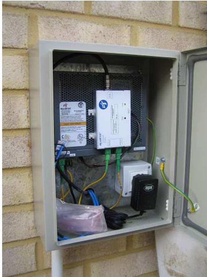
Figure 5 – A typical FTTP ONT installation. At BES in WA (Source: Opticomm)
