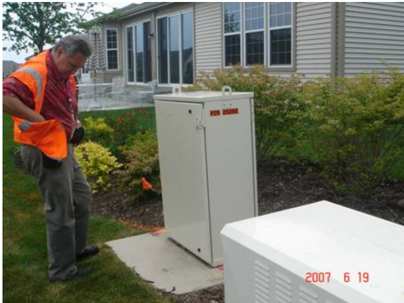
Figure 2 – Brownfield Centralised Splitter and Distribution Cabinets – FDH (Source: ADC)
