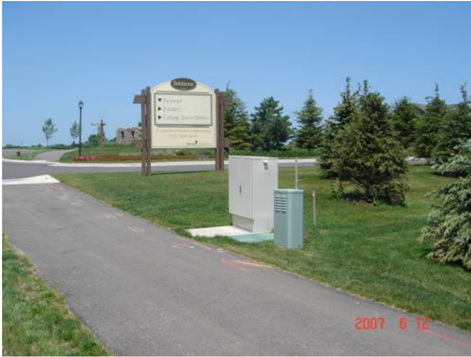
Figure 3 – Greenfields FDH Cabinets (Source: ADC)
