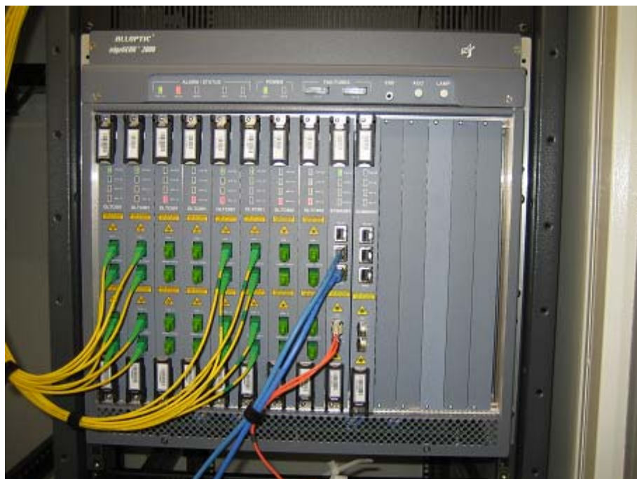
Figure 6 –Head End Equipment installed at BES in WA (Source: Opticomm)
