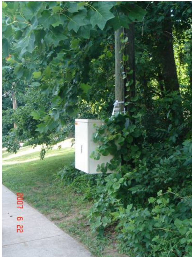
Figure 4 – Fibre Distribution Hub Pole Mount (Source: ADC)
